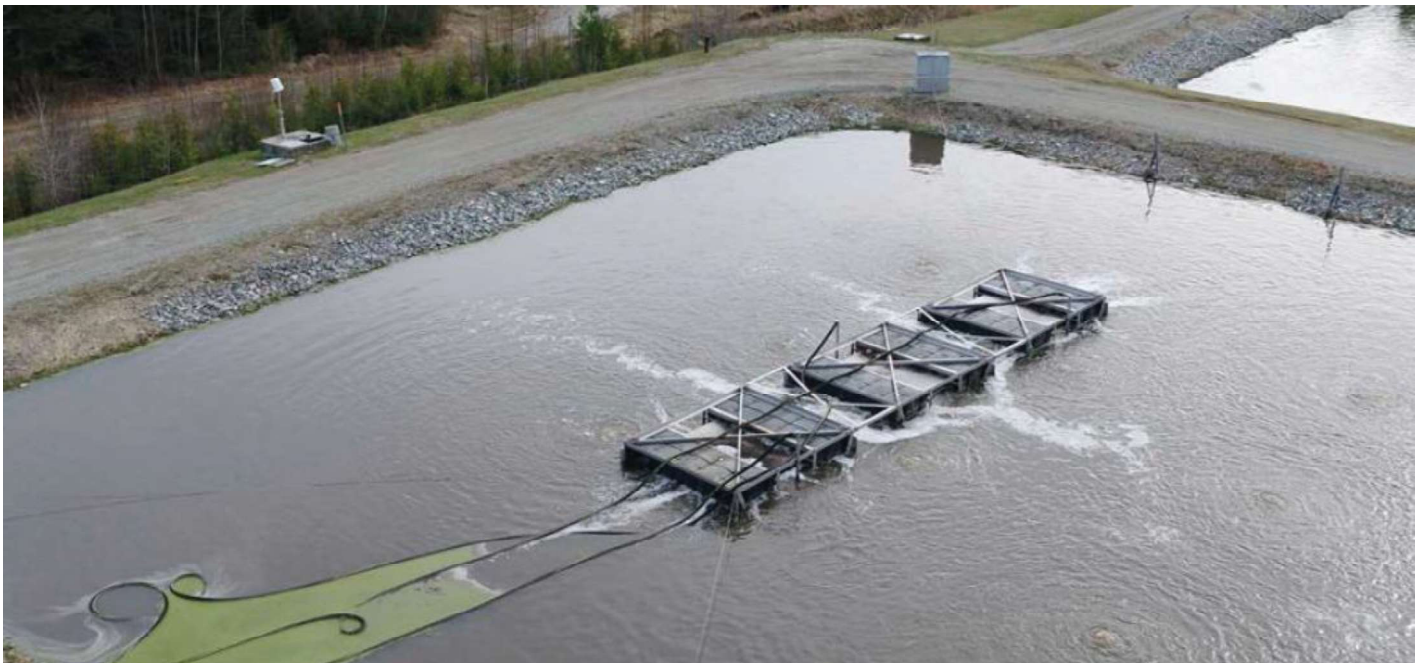
Completed installation of ECOFIXE at Ascot Corner
